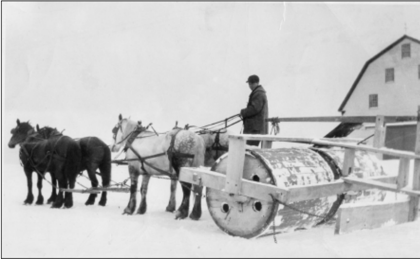
Snow roller, Caribou, 1930. The use of the snow roller was one example of changing ideas about better road maintenance at the end of the nineteenth century. A snow roller was an improvement over a snowplow as it packed down the snow on the roads, creating a wide, hard, smooth surface. Courtesy of the Caribou Public Library, Caribou, Maine.
