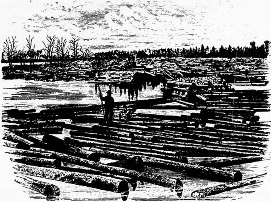
Logging dams and canals left a lasting mark on the Maine landscape: flooded lake shores ringed with dead and bleached timber, or “dry-ki.” In this illustration, river drivers standing on logs in a boom prepare to move the drive across a lake. Steele, CANOE AND CAMERA.
