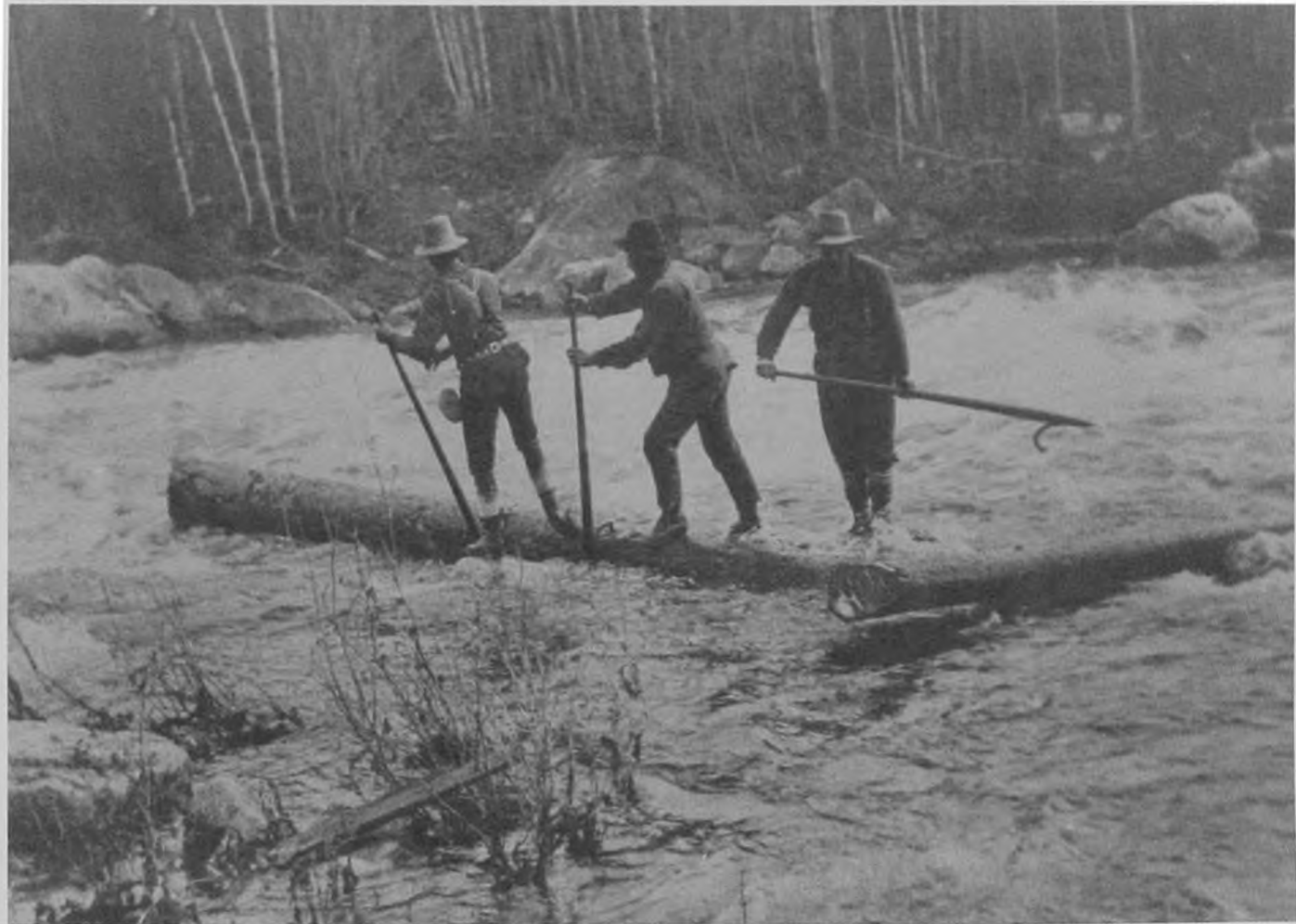
River driving required a stout heart and a talent for staying on a log in the tumbling waters of a Maine river. Each of these drivers learned the tricks of the trade as a youth and he probably endured some right of passage before gaining entry into the fraternity of men who made this dangerous business their stock in trade. Maine Folklife Center Photo #302.
