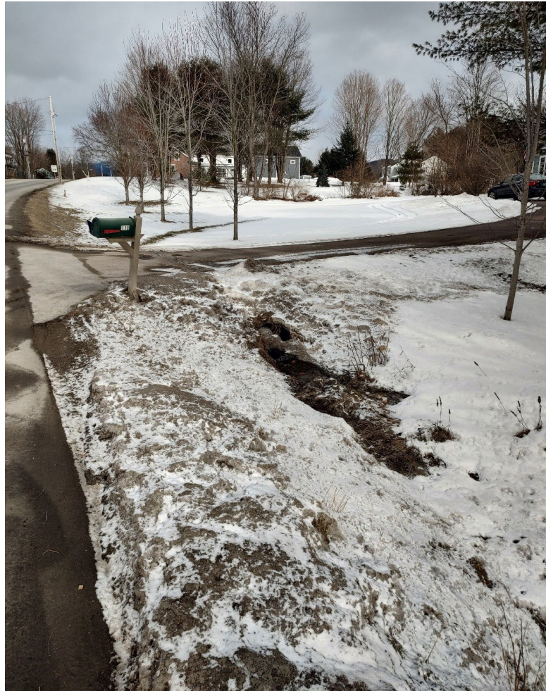
Figure 1. Daddy Falls and Curses Culvert. (Photograph taken by author).
