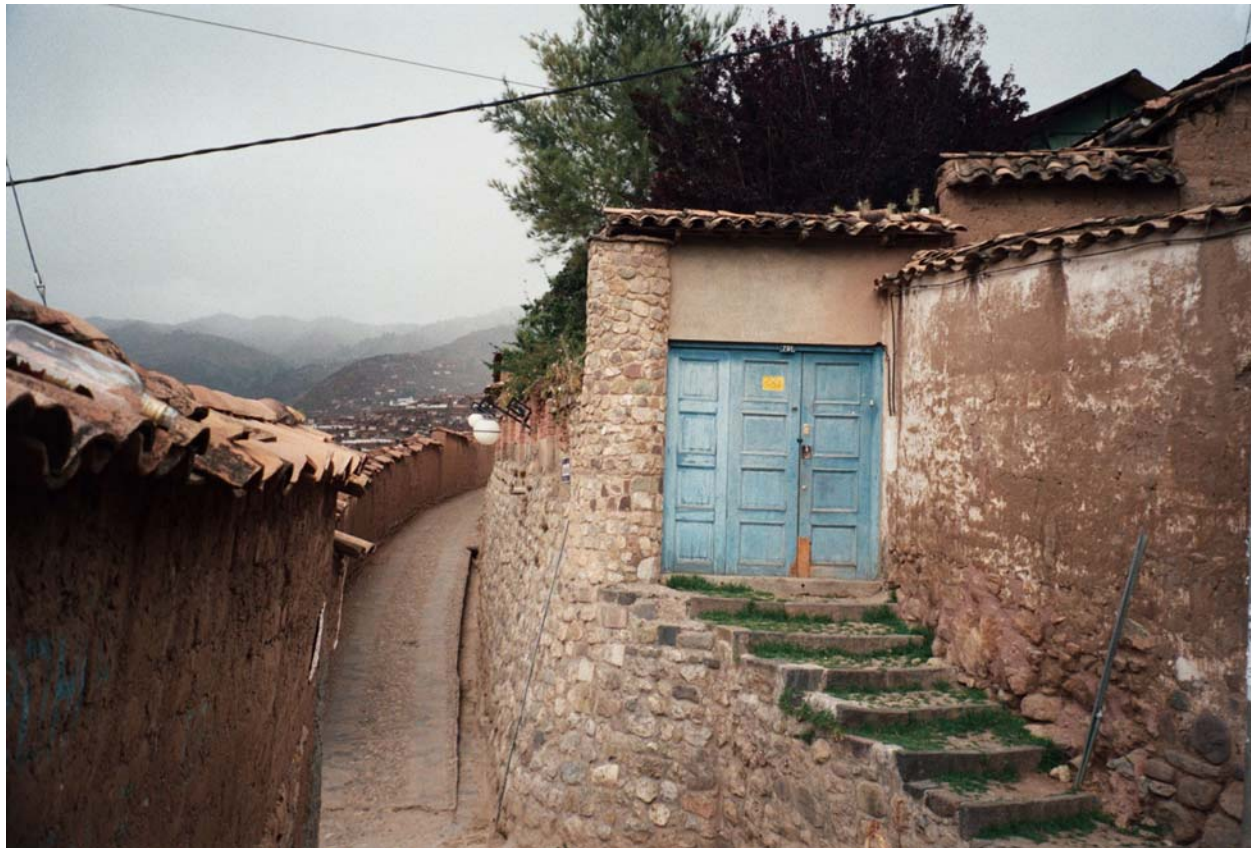
Figure 4: View of the structure at 702 Tandapata Street.
