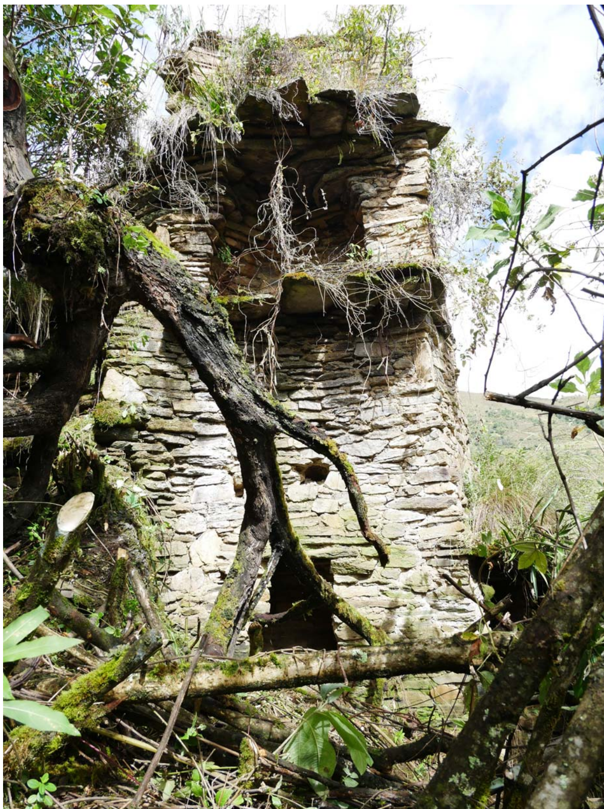
Figure 7. Multi story-building of Uchucmarca (site 10) still containing human bones (first and second levels). Note the overhanging stone platforms on the third and fourth levels.
