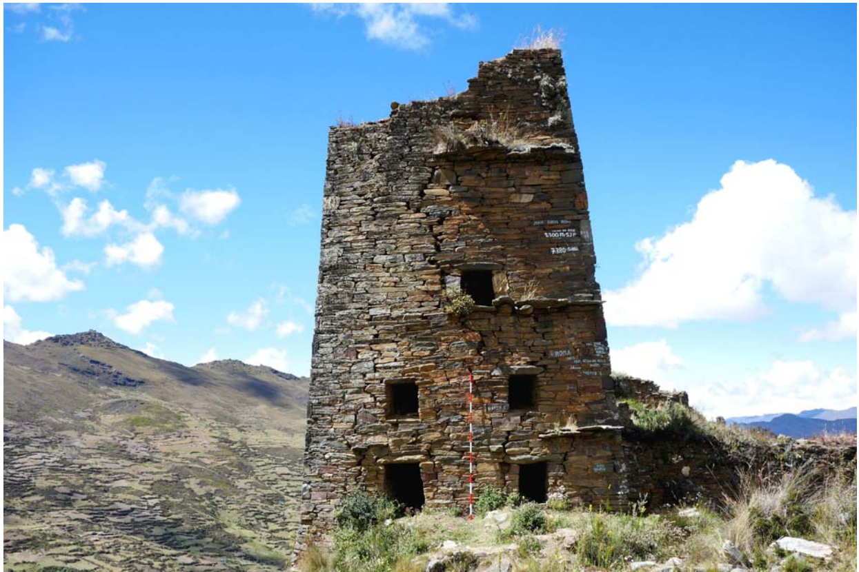
Figure 5. Multi-story building displaying overhanging stone platforms beside the windows, area I of Huata (site 16).
