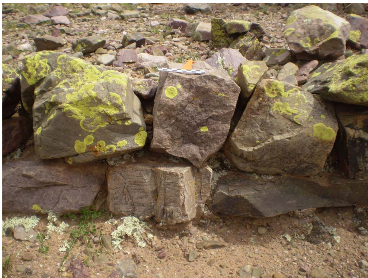
Figure 9. Blocks laid in a regular manner.
