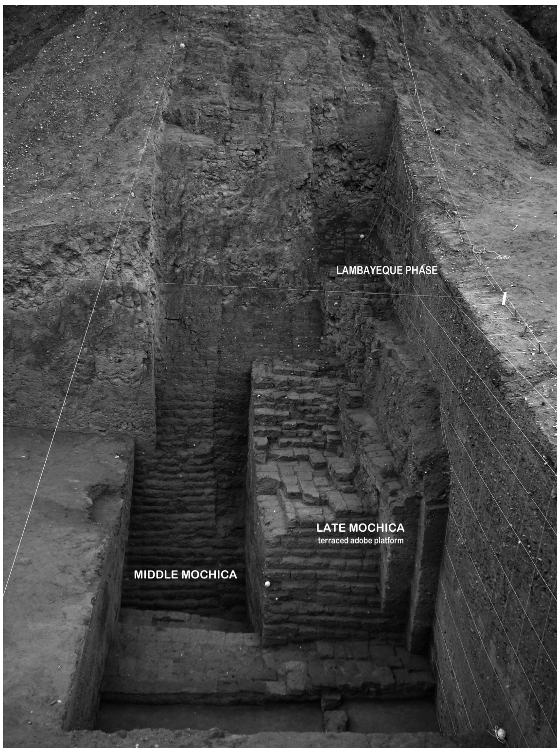
Figure 3: Late Moche buttresses built above a rubble cap on the inclined facade of the Middle Phase administrative pyramid at Sipán. Photograph courtesy of the Sipán Project.
