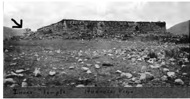
Figure 2: East (front) and south (viewer's left) sides of ushnu platform, Huánuco Pampa, 1922. Arrow marks rough construction made from outer casings of the staircase. Photo CSA46495 by John Todd Zimmer courtesy of the Field Museum.
