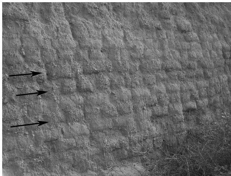
Figure 17: A section of the north wall of Compound IV, Farfán. Note layers of bricks (indicated by arrows) with greater amounts of rock inclusions than adjacent layers.
