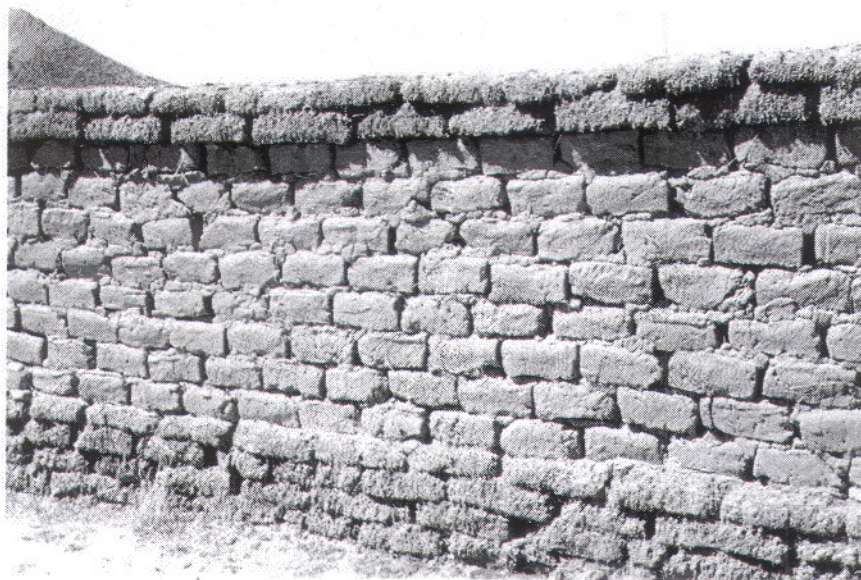
Figure 9. View of the wall surrounding the school at Yanaoqo. This 2 m high wall was built of adobe and mortar on a foundation of ch'ampa layers set at ground level for protection against ground moisture, and was capped with ch'ampa layers above to protect against rain.
