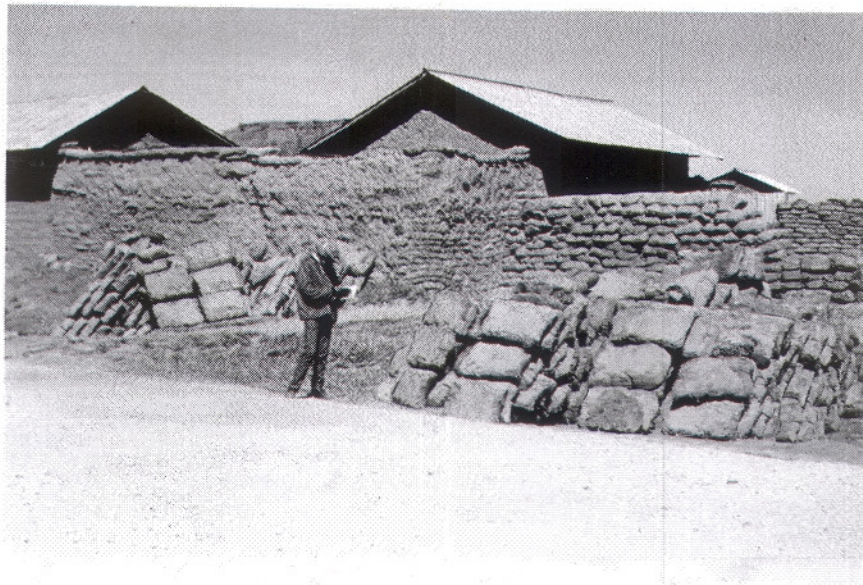
Figure 8. Blocks of ch'ampa brought from Yanaoqo Pampa and stacked near the site where a putuku will be built.
