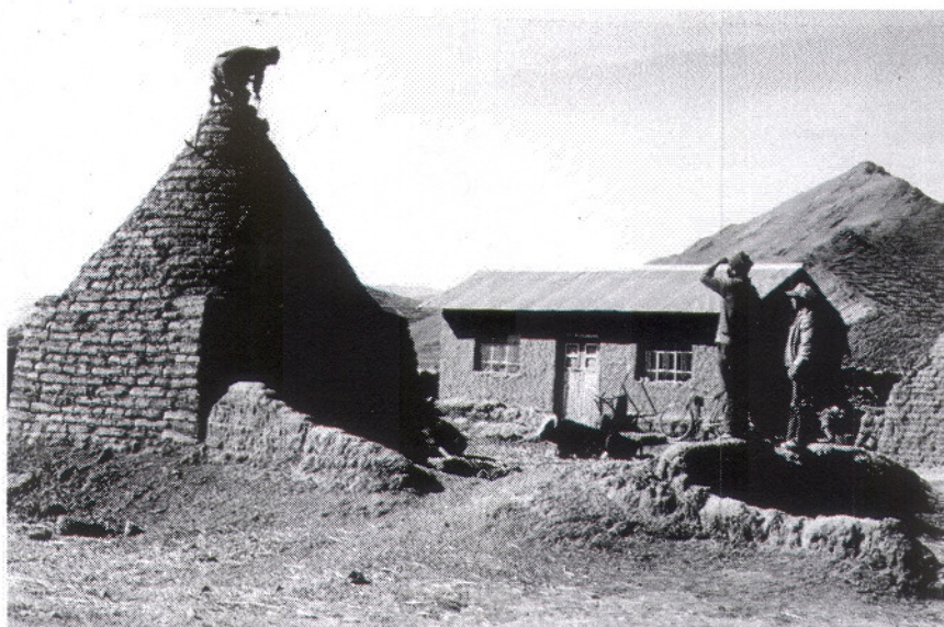
Figure 10. View of a household cluster in Yanaoqo composed of a putuku , a small corral on the left, and a gabled structure. The gabled structure is built of adobe with stone foundations which extend about 40 cm above ground. The roof is built of corrugated iron sheets, the door is carpentry made, and the glass windows have metal frames. The structure being built is a putuku .
