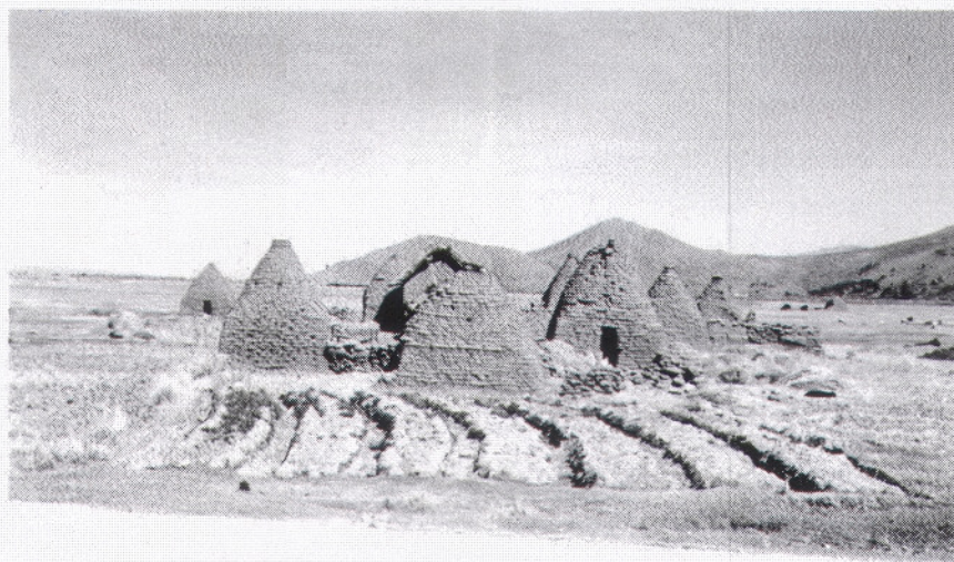
Figure 15. An abandoned household cluster in Yanaoqo. Note the doors closed with ch'ampa blocks, and the collapse of the entryway and apex portions.
