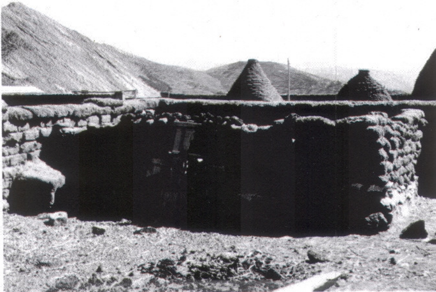
Figure 19. The northern portion of Mariano's household cluster. A corral attached to the northwest corner walls, in which two of the walls are built of two layers of irregular stone at the bottom followed by ch'ampa layers on top.
